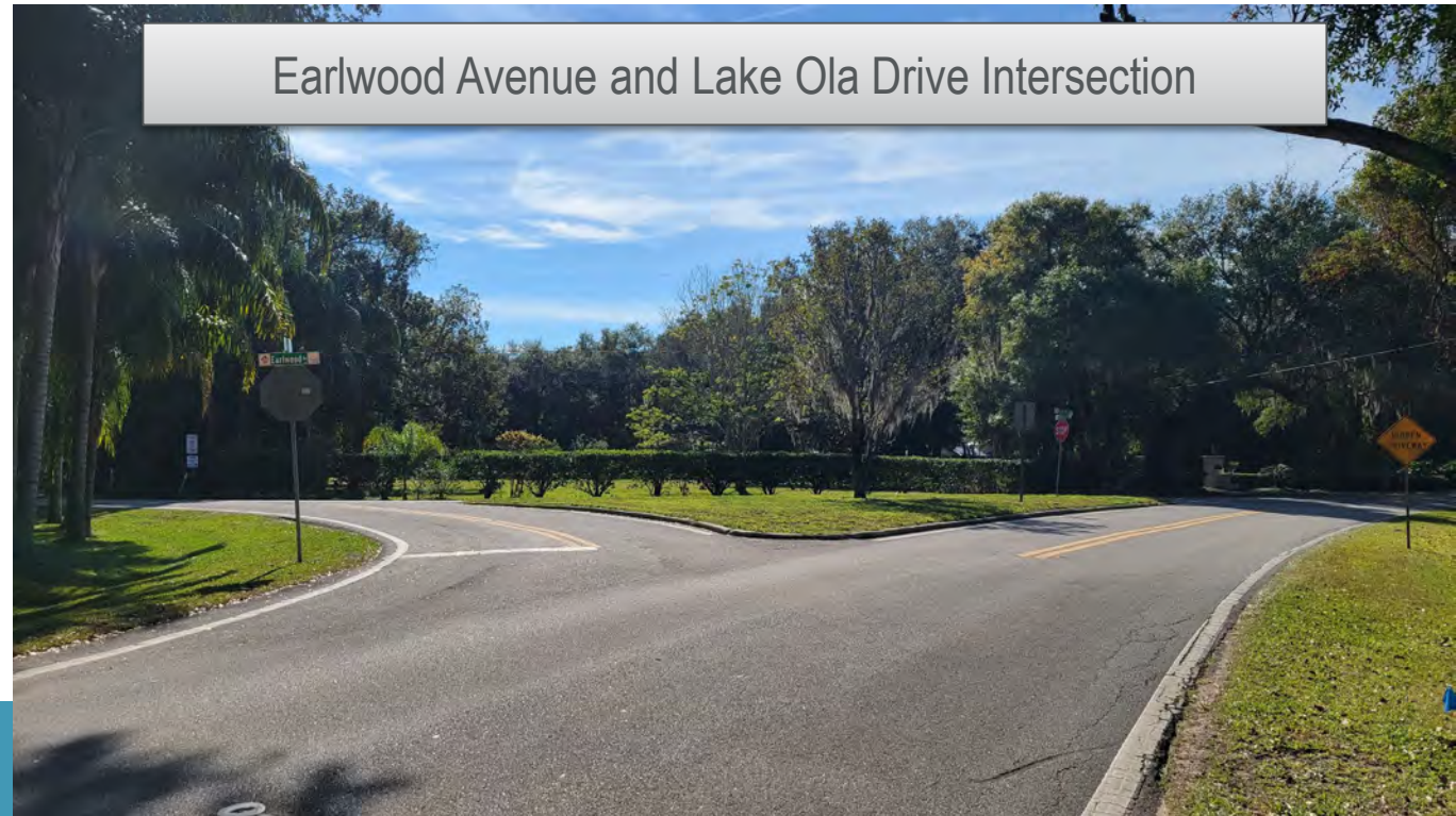
Earlwood Avenue and Lake Ola Drive Intersection
